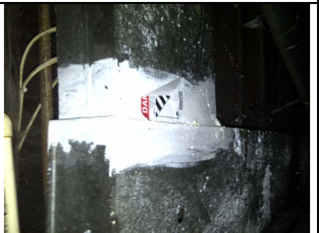
6: Assumed ACM ducting joint compound in the basement.
