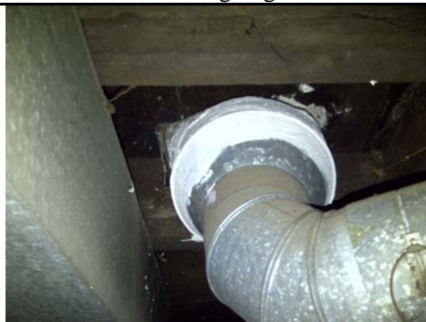
5: Assumed ACM piping in the basement.
