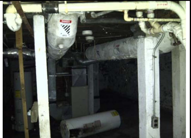
4: Assumed ACM piping in the basement.
