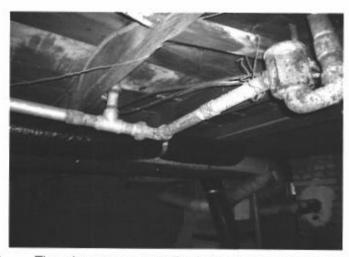
There is an open waste line in the basement near the laundry tub. This could allow sewer gases into the building interior. This should be repaired.
