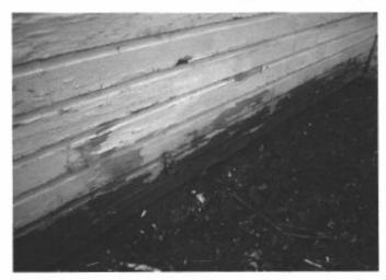
The paint coating on the garage walls and trim is deteriorated. Paint and other coatings are a barrier on surfaces to protect the substrate from deterioration due to sunlight and weather elements. See house exterior comments for recommendations.
