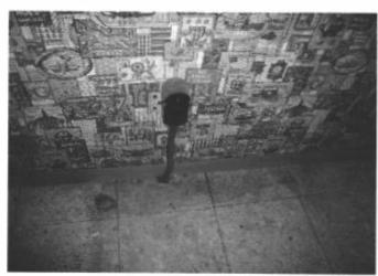
Junction box covers or knockouts are missing. Fully enclosed junction boxes are required for fire and mechanical protection. Adding covers is recommended.
